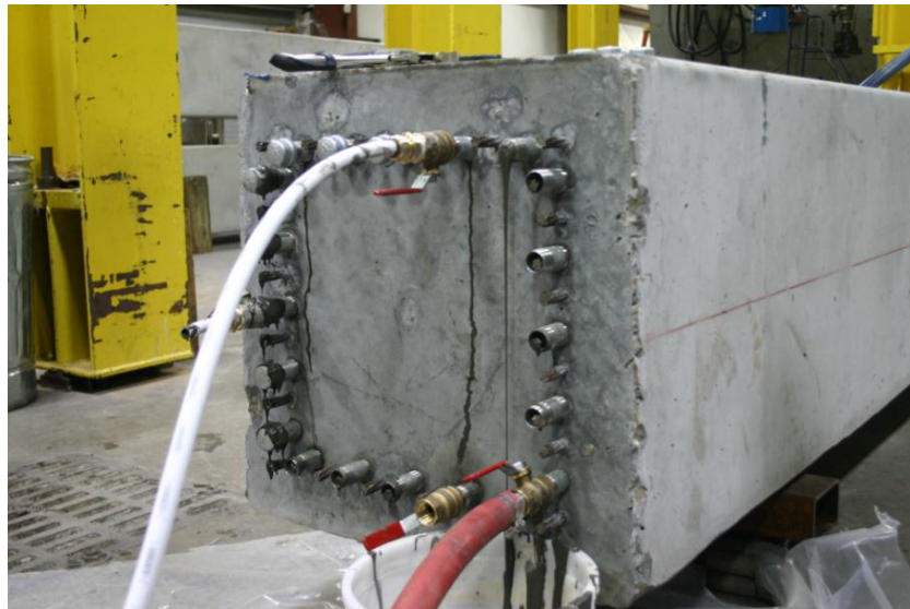
Figure 4.10 Grouting post-tensioned strand ducts.
