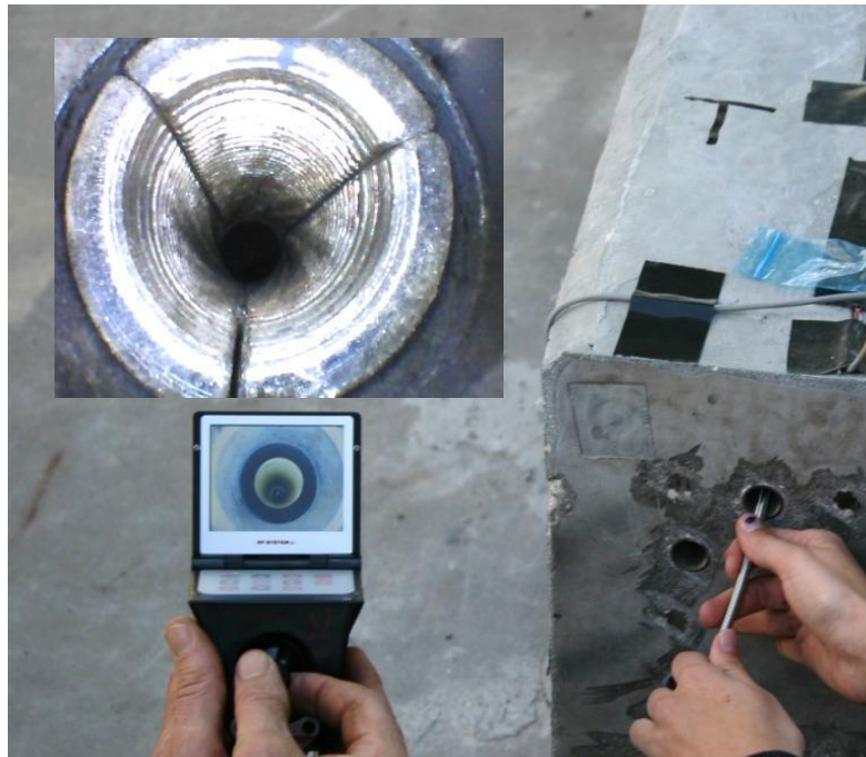
Figure 3.10 Inspection of ducts using borescope.
