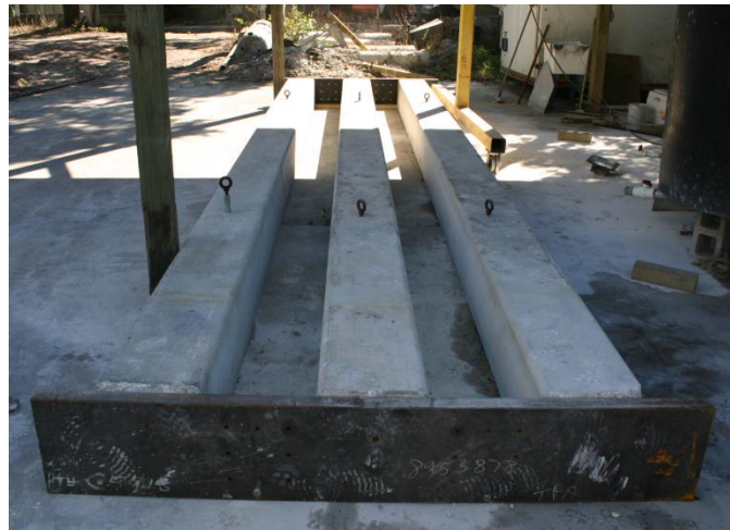
Figure 3.2 Casting bed for test piles.
